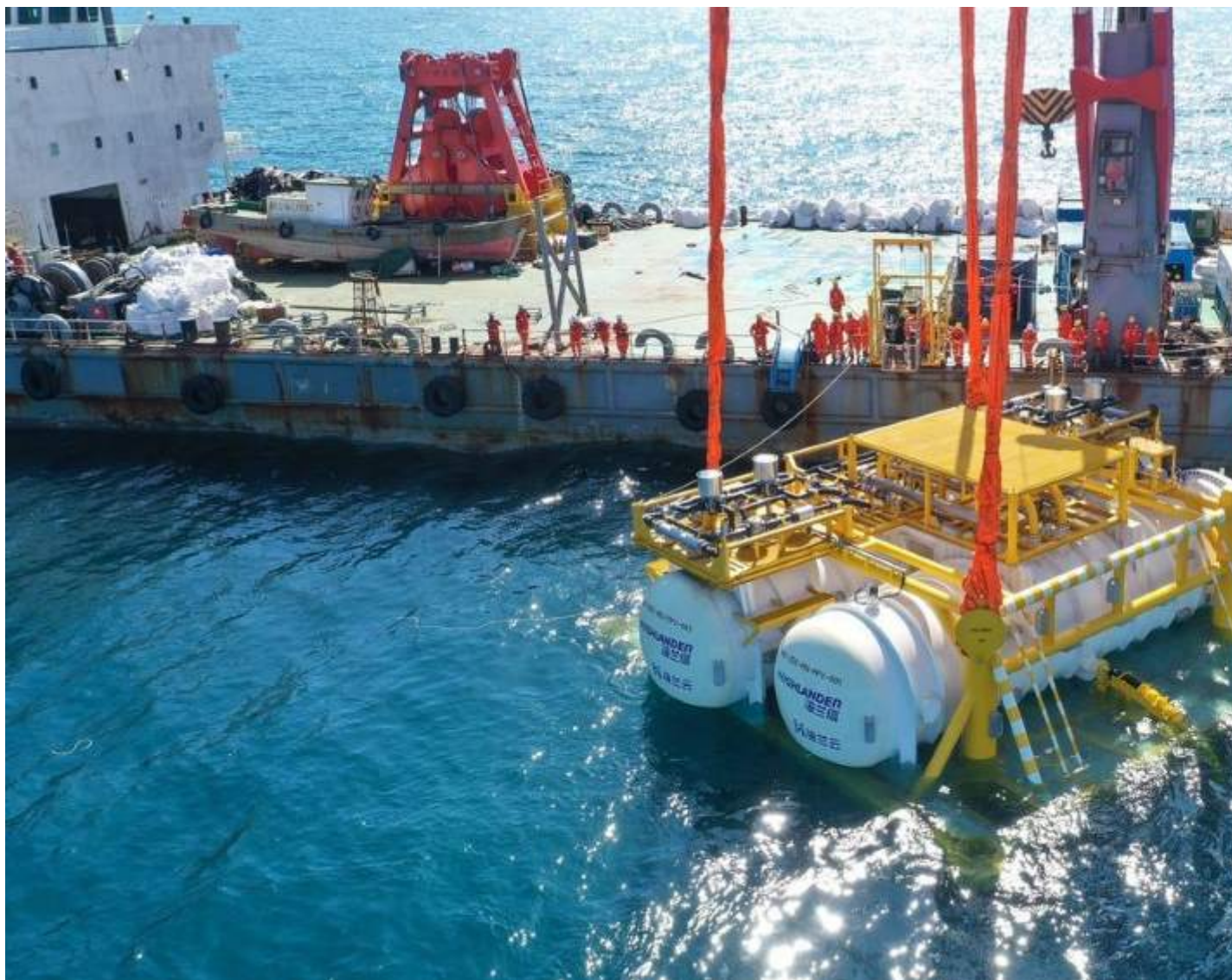
Figure 5: The first module of the Hainan Undersea Data Centre
